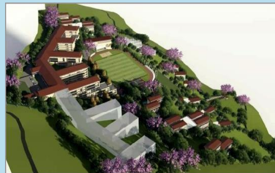
Permanent campus under construction at Temi Tarku, South Sikkim
